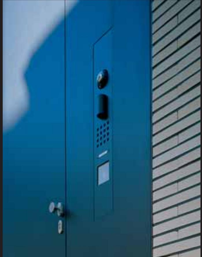
The mounting level is recessed so that the control level fits exactly flush with the surrounding surface. Forward projections are only present where the function demands them – as for the video camera and the spot lighting. Like the surrounding door panel, the system pictured is coated with the extremely durable and dirt-resistant Duraflon.
