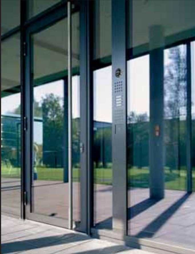
The panel installation, the second option for glass mounting, positions the communication technology between two glass elements. Without using an additional frame, the Steel panels become an integral part of the glass façade. The uniform paint finish further highlights the homogeneous impression.
