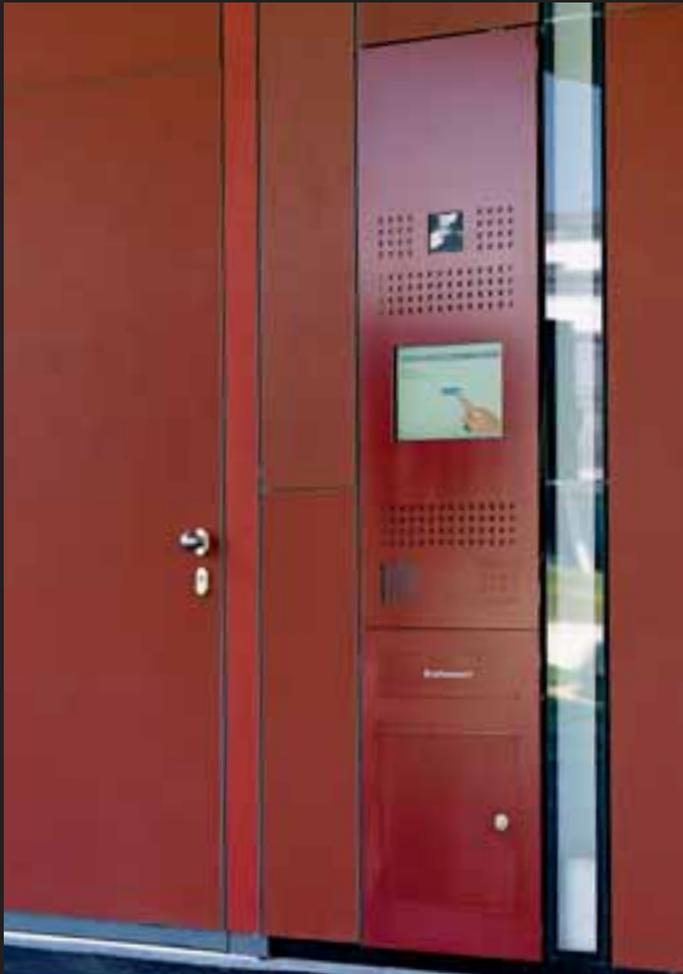
The communication terminal is based on an industrial PC optimized by Siedle to achieve extreme operating security. It performs all the functions of a door station including access control by code lock and connection to the public telephone network. Furthermore, it opens up the entire world of PC-aided information and access to the Intranet or Internet.
